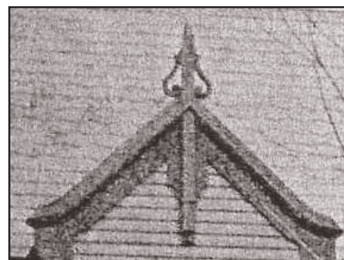
Detail from historic photo of acroteria.
